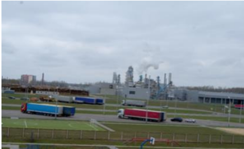
Parking for trucks Commissioning - July 2013
