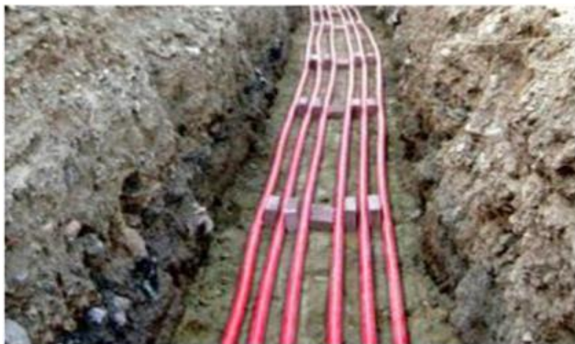
Communication network of 17.37 km total length Commissioning - August 2013
