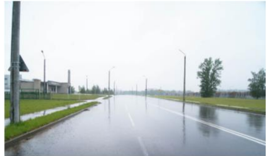
Auto roads Commissioning - July 2012 Length - 0,43 km
