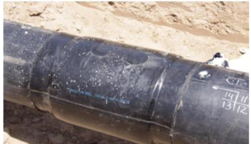
Heating network of 0,84 km length Commissioning - August 2013
