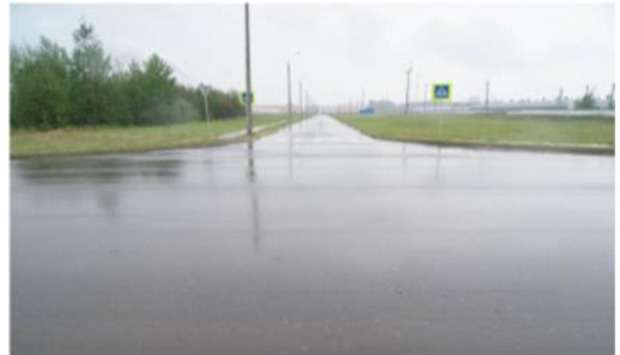
The road network The total length - 5,1 km Commissioning - August 2013
