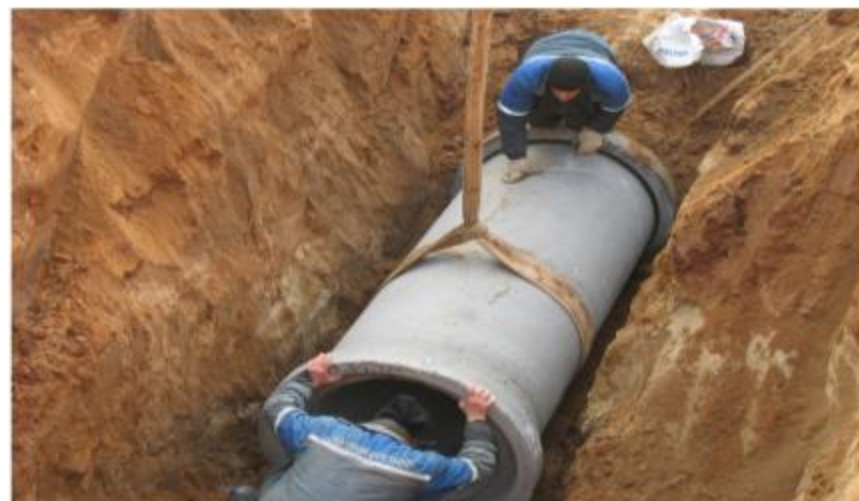
Sewage system Commissioning - August 2013
