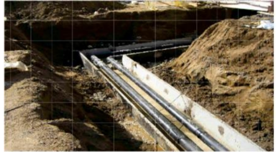
Technical water supply pipeline with a length of 1,926 km Commissioning - June 2015
