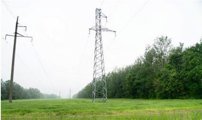
Power transmission line 110 kV Commissioning - May 2012 Length - 2,19 km
