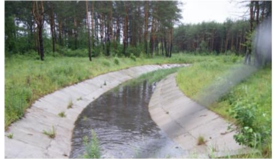
Drainage ditch Commissioning - July 2013
