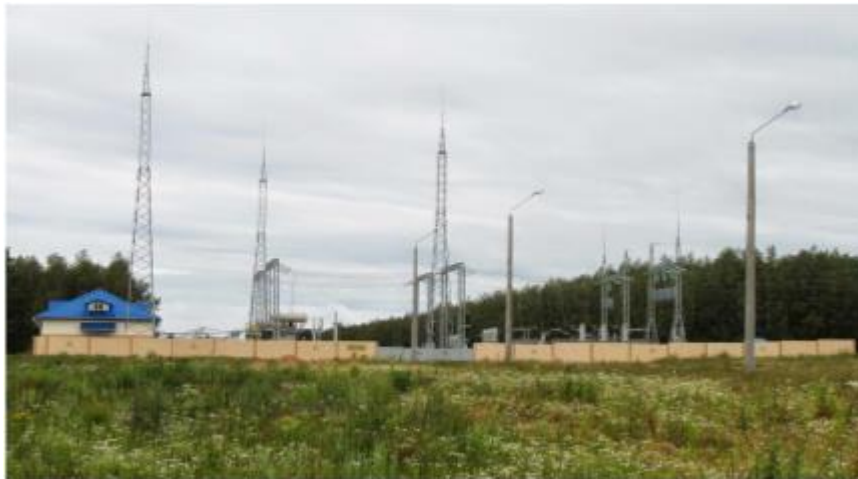
110/10 kV substation "Industrialnaya" Commissioning - August 2012 Two transformers of 40 MW each one
