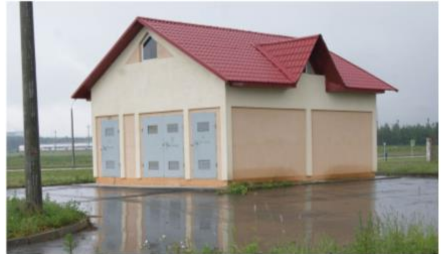
Transformer substation with a capacity of 250 kW Commissioning - August 2013
