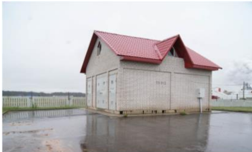
Transformer substation with a capacity of 150 kW Commissioning - August 2013
