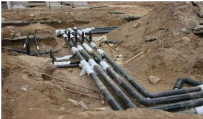
Drinking water pipeline The total length - 12,508 km Commissioning - August 2013
