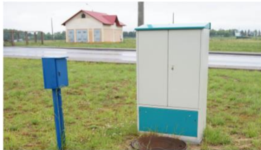
Fiber-optic communication lines Commissioning - August 2013
