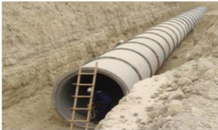
Rainwater drainage The total length - 6,67 km Commissioning - July 2013
